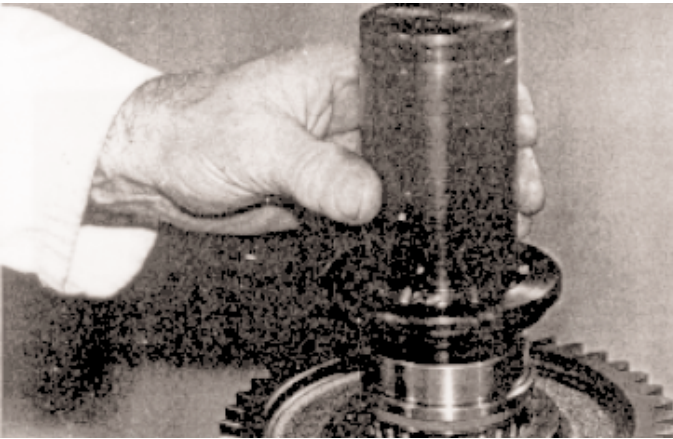
18. Take the heated inner track of the mainshaft rear bearing and fit it over the shaft, flange innermost against the spacer. Use a soft drift or flanged driver if necessary to ensure that the bearing is fully home against the shoulder.
