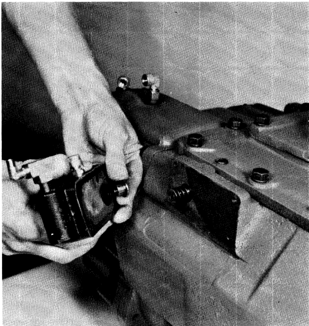
178. Installing the alignment sleeve in air valve.
